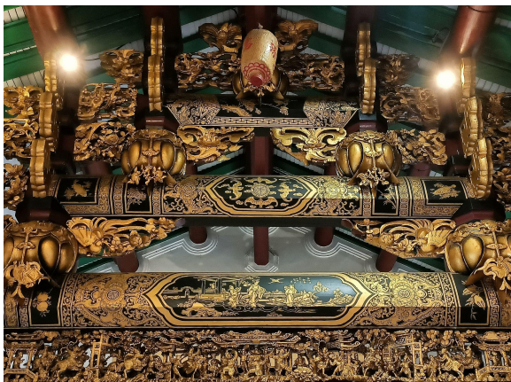
Figure 15 Temple trusses that stacked one atop another, 2022.
